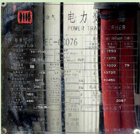
OIL TRANSFORMER 1500KVA & 2500A MSB c/w Capbank
