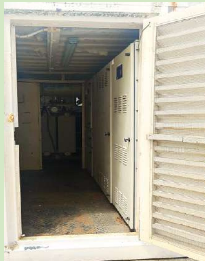
OIL TRANSFORMER 1500KVA & 2500A MSB c/w Capbank
