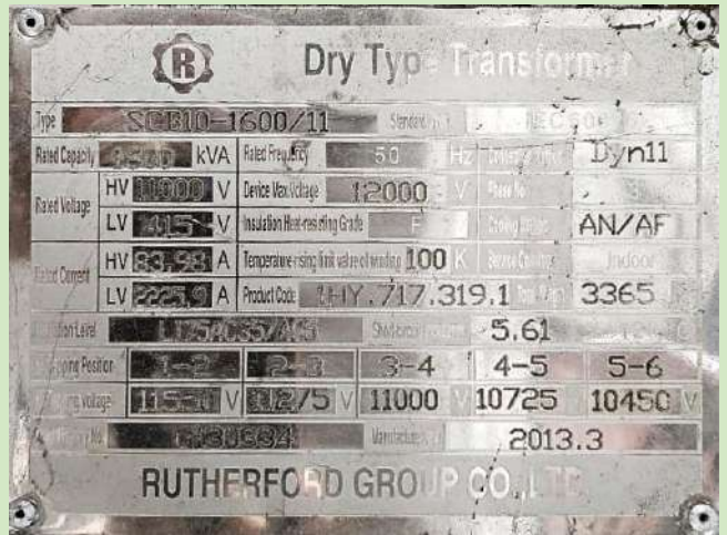
CAST RESIN TRANSFORMER 1600KVA
