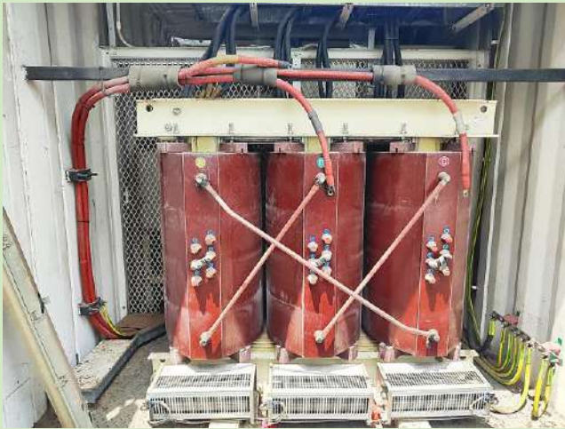
CAST RESIN TRANSFORMER 1600KVA
